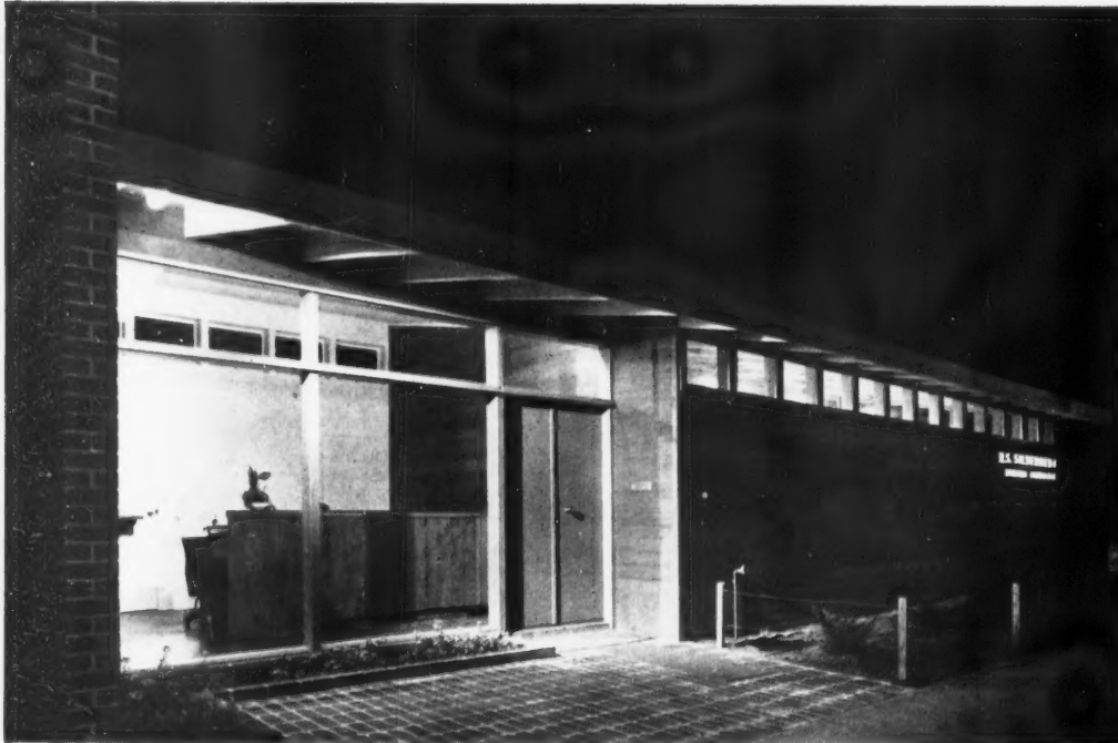
13, the office seen from the street. Timber walls are faced with stained redwood siding.
