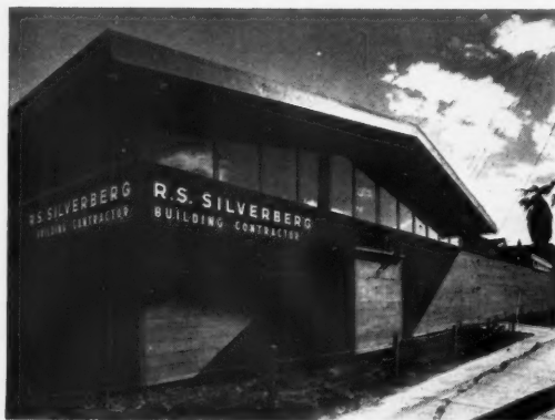
15 & 16, interior and exterior of the workshop in which minor mill-work is done. In 16, the flush doors to the yard can be seen beyond the workshop.
